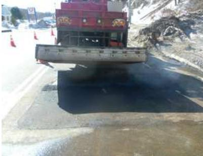
Since crews are putting hot asphalt onto hot asphalt, they can work in the snow, with no cold joints.
